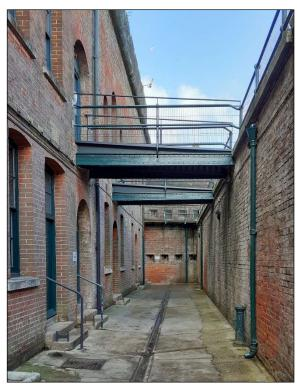
The completed bridges are finished with a familiar conservation architect's technique. The new materials are rendered in a modern gunmetal grey finish while the original materials are painted in a traditional dark green.
